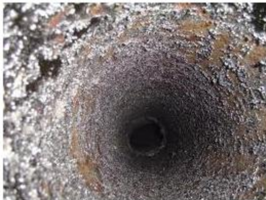
Flue before chimney sweeping
