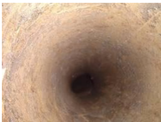
Flue after chimney sweeping
