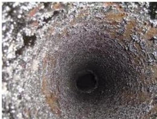
Flue before chimney sweeping
