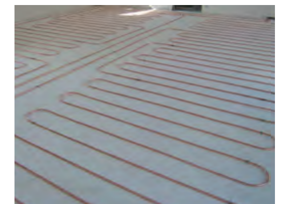
3 _ Spiral: ensures that heat is distributed in a uniform manner. It is recommended for regular surfaces.
