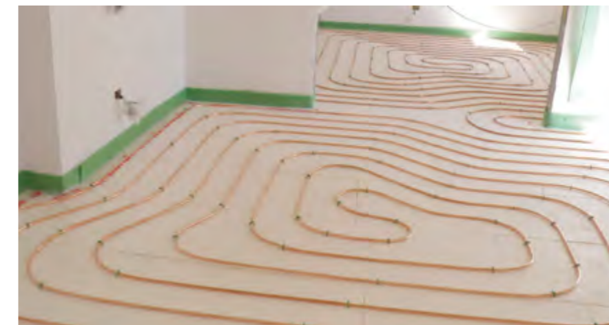
3 _ Spiral: ensures that heat is distributed in a uniform manner. It is recommended for regular surfaces.
