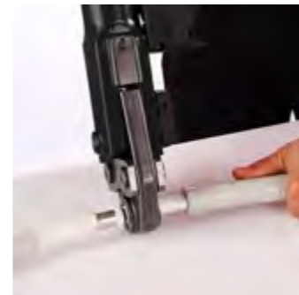
Press-fitting (Alternatively you can use compression or quick coupling solutions)
