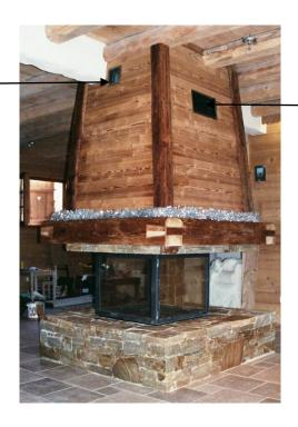
Clean the inside of the installation using a vacuum cleaner or brush in order to eliminate any dust deposits causing carbonization of dust (dirt around the hot air outlets and on the ceiling) at the start of the heating season and once during the heating season.
